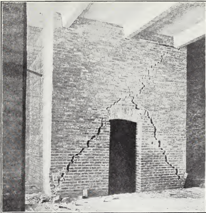
A. EARTHQUAKE CRACKS IN WALL OF VAULT, CALIFORNIA CASKET COMPANY'S BUILDING, SAN FRANCISCO.
